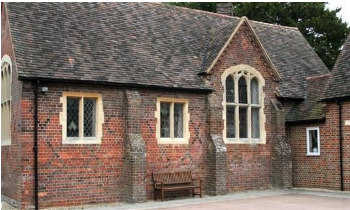
Buckland Village Hall
