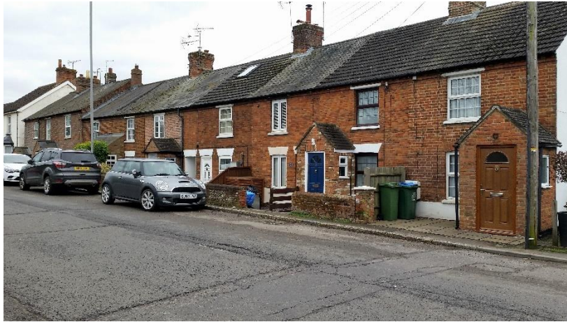
Buckland Wharf Cottages
