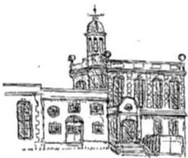
DANCERSEND PUMPING STATION
